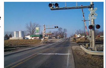
Railroad Crossing with Cantilever Flashing Lights and Gates
