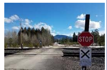
Multiple tracks Railroad Crossing
